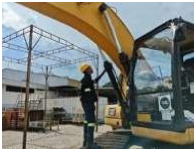
Gambar 4. 1 Pengecekan Cylinder Boom
